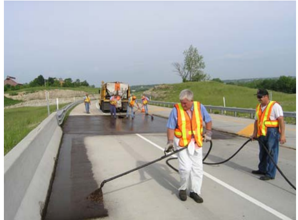
(2) In-Deck Seal Application
