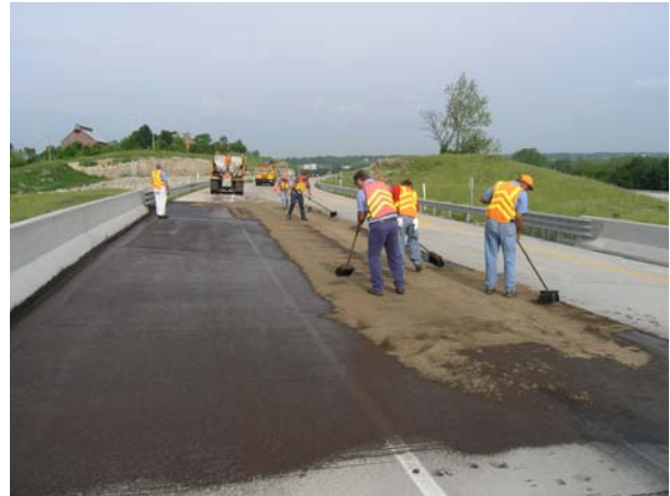
(4) Sanding In-Deck Seal
