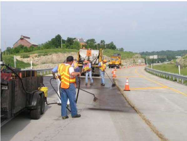
(3) In-Deck Seal Application
