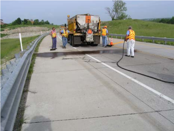
(1) In-Deck Seal Application
