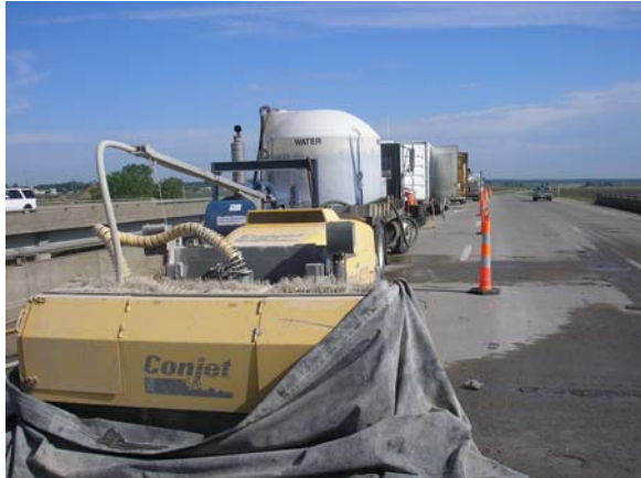
(1) Hydro Demolition Set Up for Spot Repair
