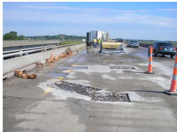
(4) Results of Hydro demolition for Spot Patching
