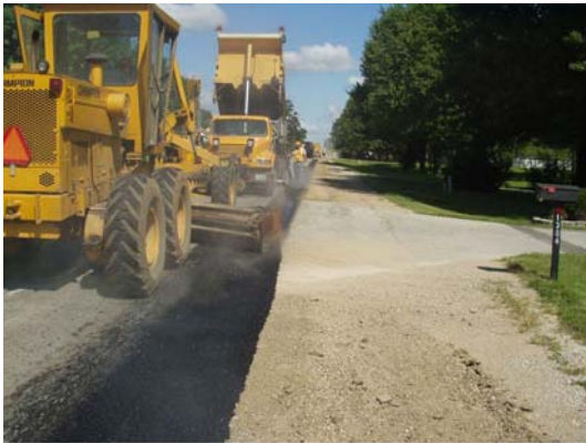
(7) Hot-Mix Lay Down
