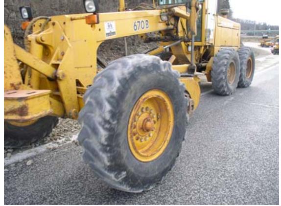
(14) Blading 2" Aggregate with Motograder
