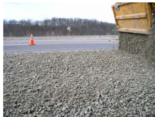
(12) Applying 2" Aggregate to Outside Edge of Shoulder
