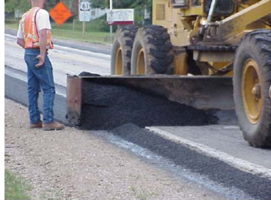
(8) Box Blading Hot Mix Asphalt
