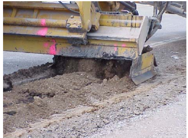
(4) 2' Roto Grader (Back View)
