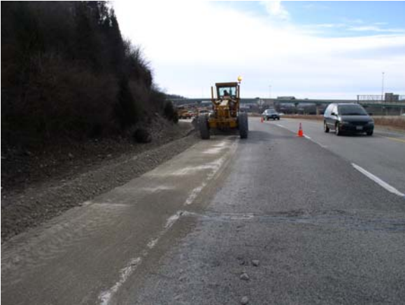
(15) Blading 2" Aggregate with Motograder
