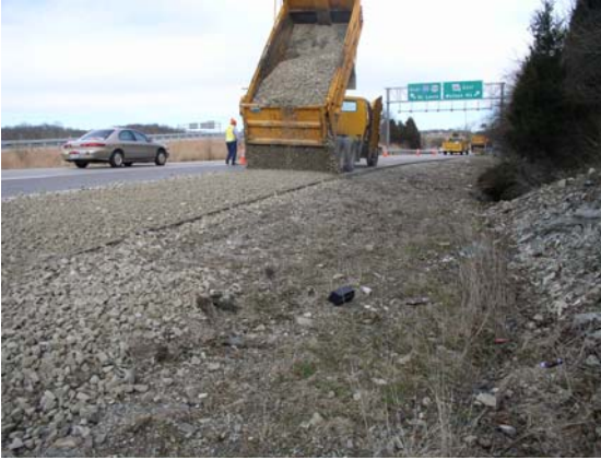
(13) Applying 2" Aggregate on Shoulder
