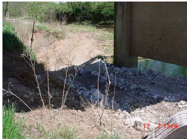
(10) Preliminary Grading for Gabions
