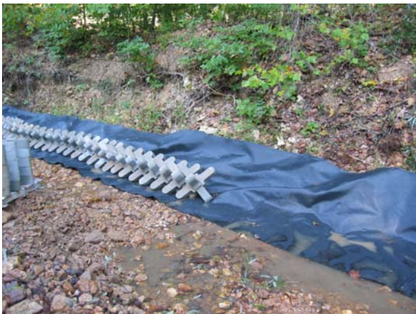
(5) Ajax Installation with Silt Blanket
