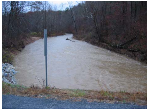
(2) Indian Creek – Upstream Full Flow Condition
