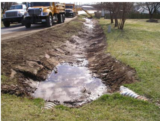
(5) Graded Culvert Ditch
