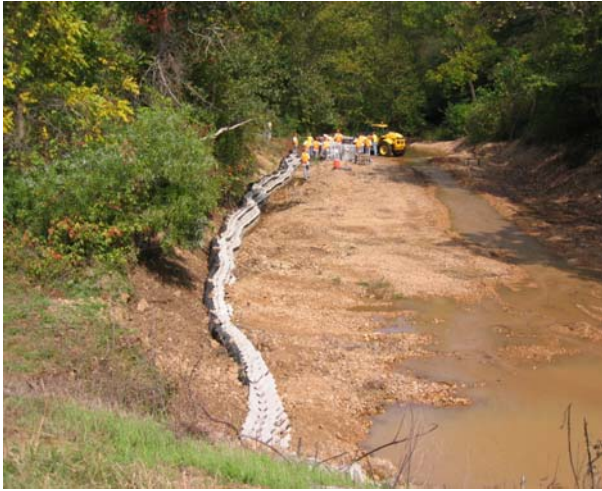
(7) Completed Installation of Ajax Blocks
