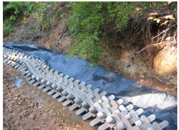
(6) Ajax Installation - Continued
