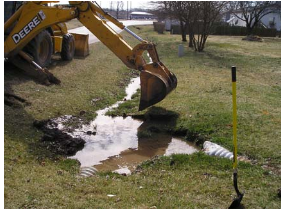
(2) Digging out Culvert Ditch
