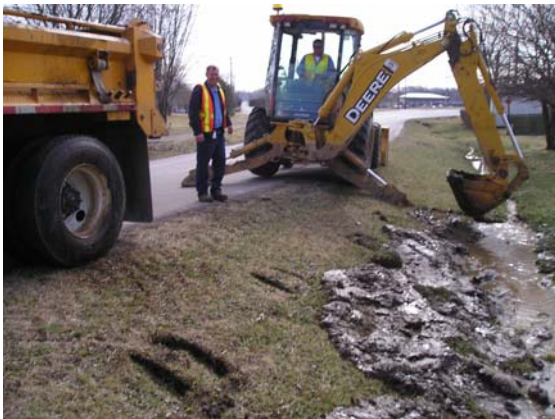
(3) Digging out Culvert Ditch
