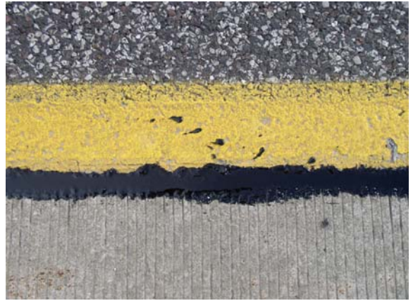
(8) Completed joints after filling:
