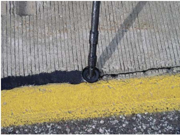
(7) Close up of wand filling the joint
