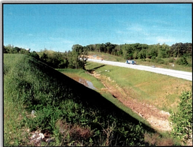
Figure 6: Permanent detention basin on Route 54 expressway.
