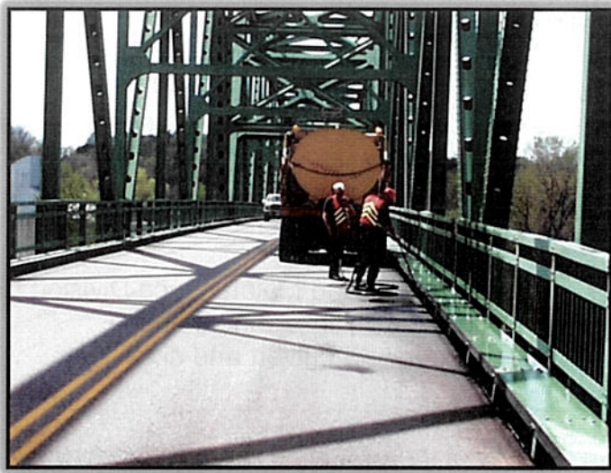
Figure 5: Street sweeping and bridge washing.
