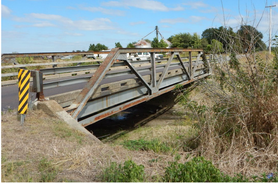
Figure 3: Bridge F0757, profile view, facing northeast
