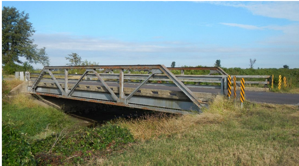
Figure 2: Bridge F0757, profile view, facing northwest
